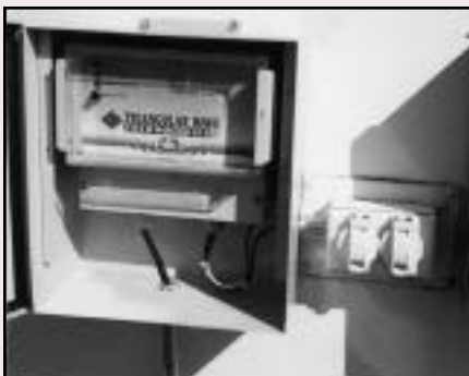
Triangularwave Technologies, Inc. Microprocessor installed in a weatherproof electrical box on the outside wall of the building.
