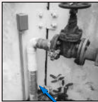
The coil is wrapped around a water pipe and protected from dirt, disturbance and moisture with weatherproof tape.
